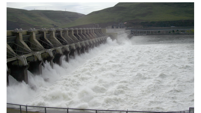
Spill helps young fish migrate past dams, but high levels increase total dissolved gas, degrading water quality.
